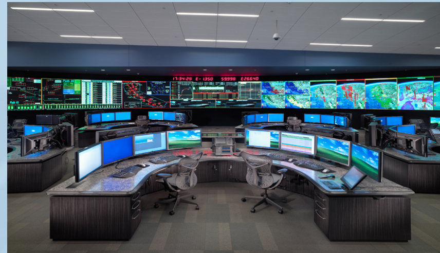
CAISO Control Room Folsom
